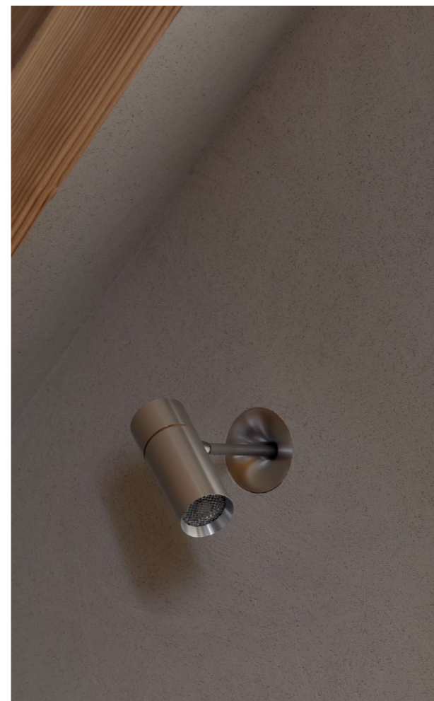
Project: Barn T | Interior design: Anne-Catherine Ramboux | Photography: Cafeine
