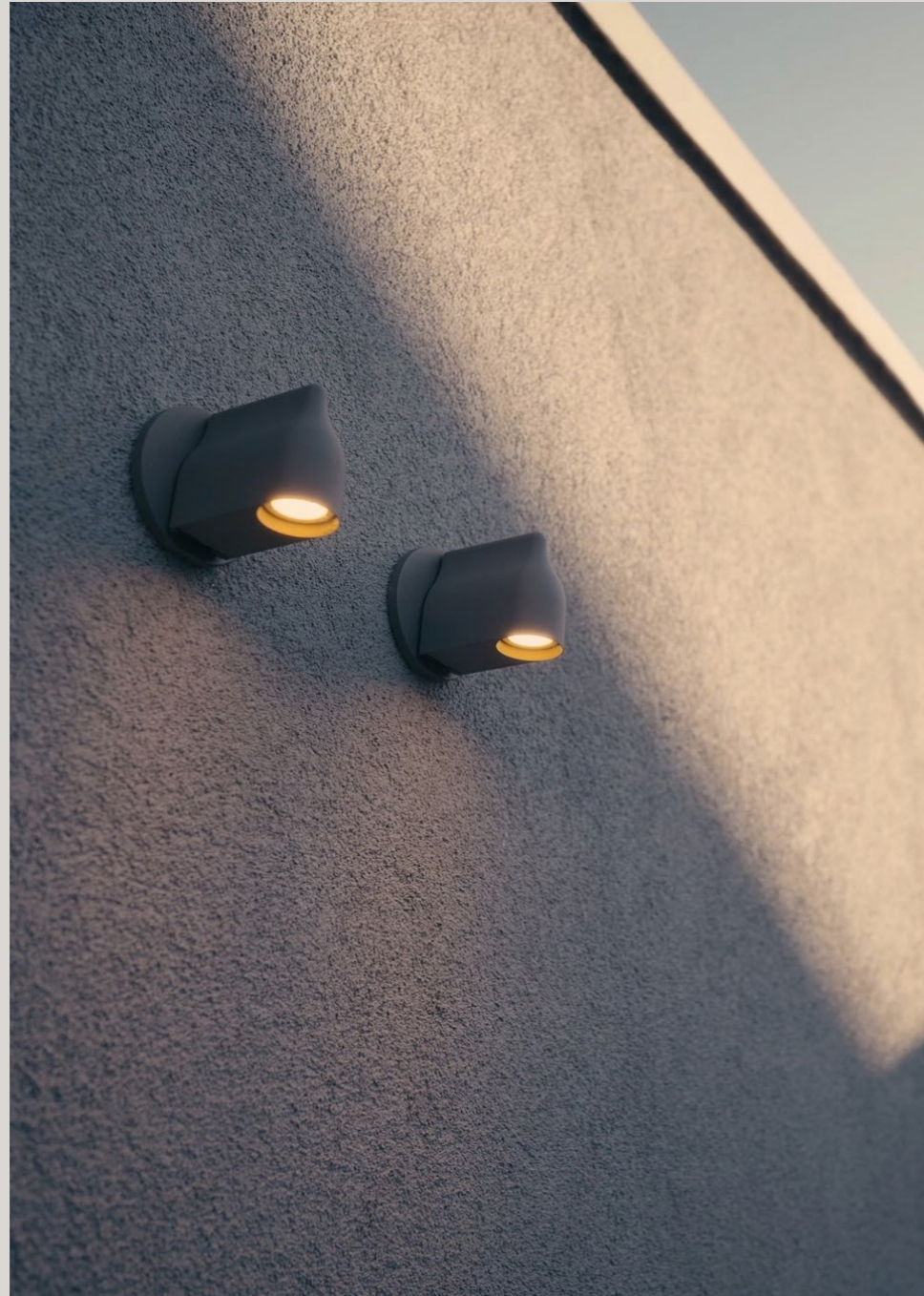
Project: Private residence | Lighting design: ONE A
