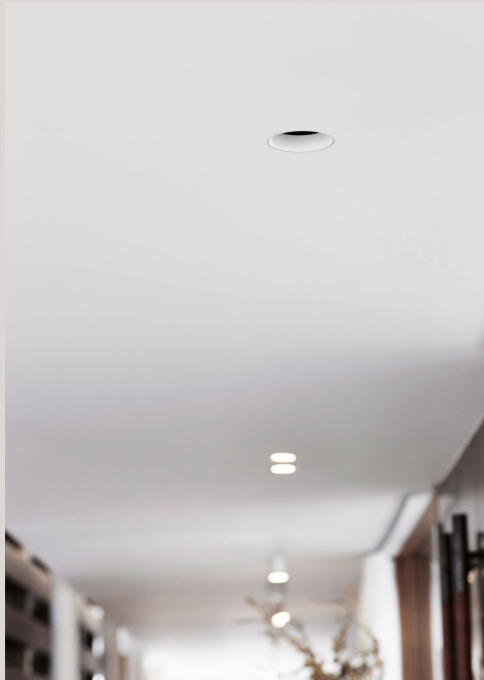
Project: Private Residence | Lighting design: ONE A
